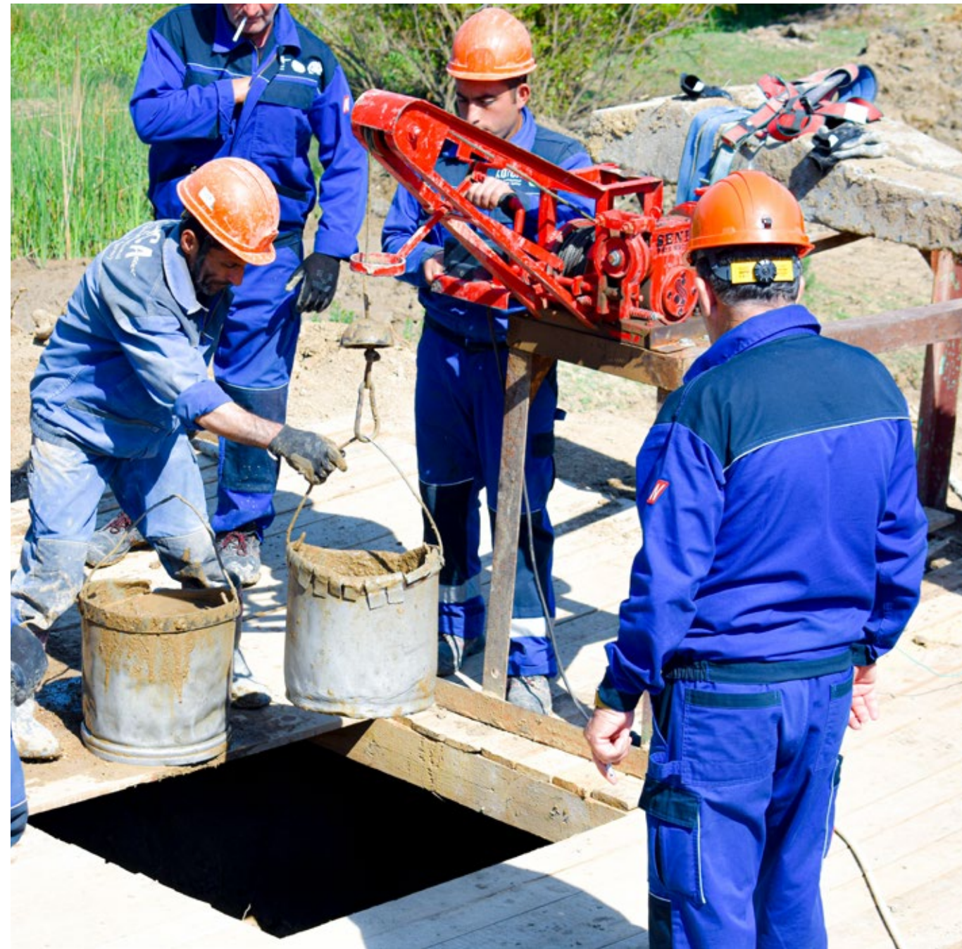
Rehabilitation works expands in ancient kahrizes- traditional, sustainable water supply systems. Photo credit: IOM/2022
