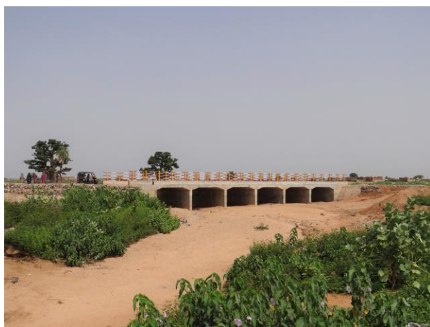
Newly built South Darfur Riyad Box Culvert ©UNOPS
