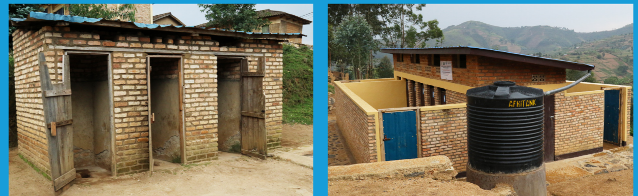
Ruhinga Early Primary School's old (left) and new (right) latrines.
