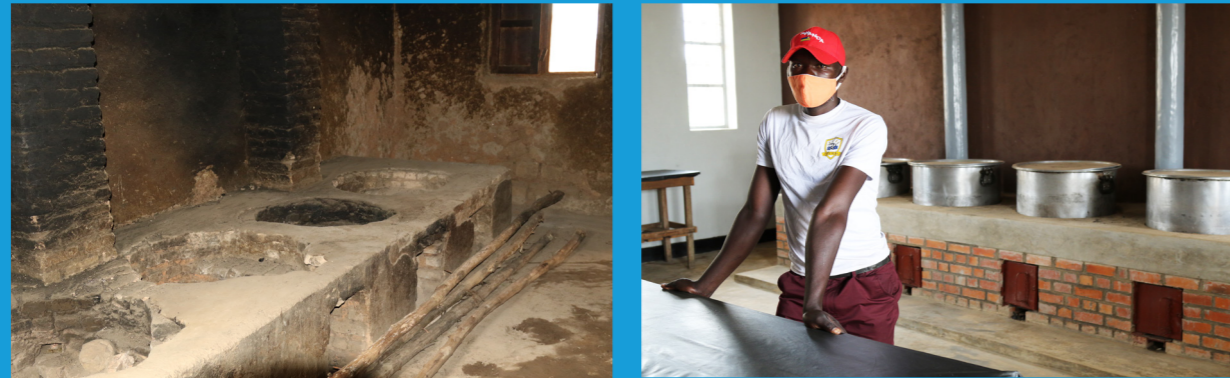
The contrast between old (left) and new (right) kitchen is stark. School cook Felicien Rwatangaro is pleased with the new facilities and looks forward to welcoming students back.
